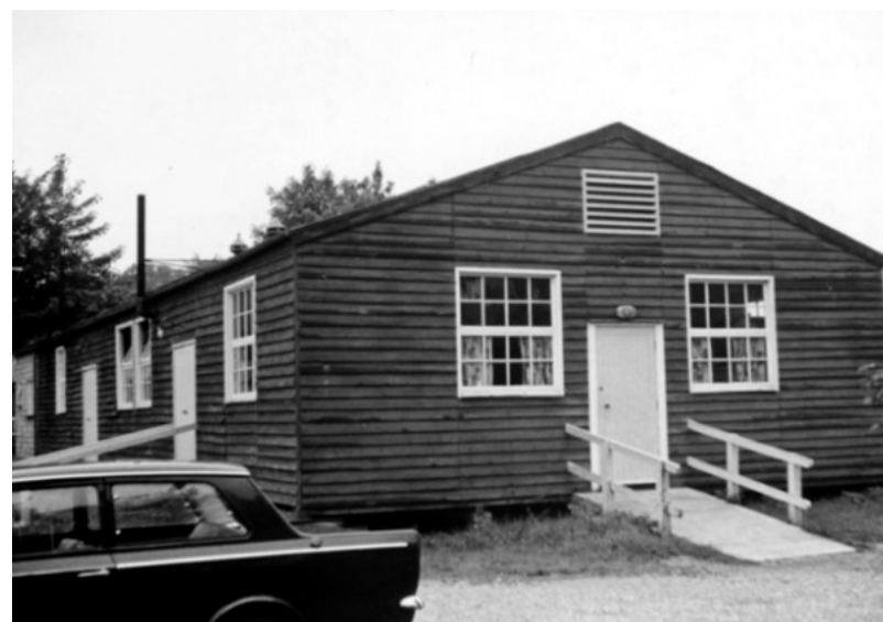
The Old Lincoln Hall. The building was previously used as the village hall at Hingham and was believed to have been brought to the site from Thetford, on the back of a traction engine, after the end of the War. (Image - Hingham History Centre Website).
